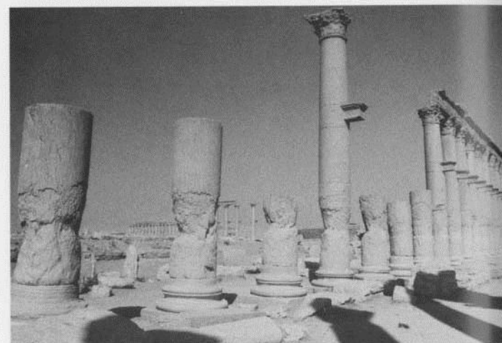
Fig. 2 The abrasion zone on the columns of the Great Colonnade.
