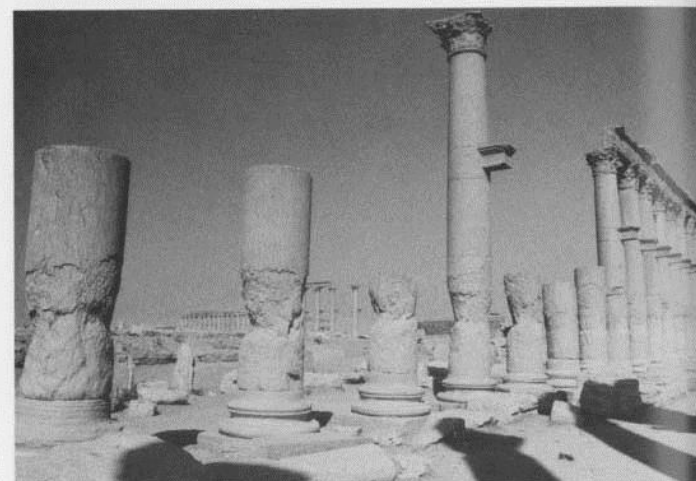
Fig. 2 The abrasion zone on the columns of the Great Colonnade.
