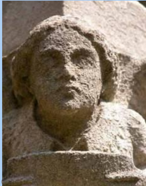
Church carving showing effects of hydrolysis
