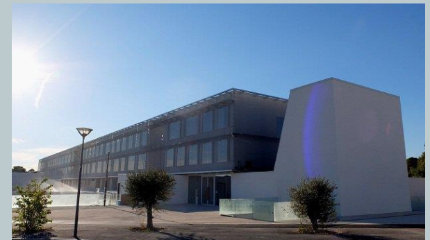
LMA at Château-Gombert Campus
