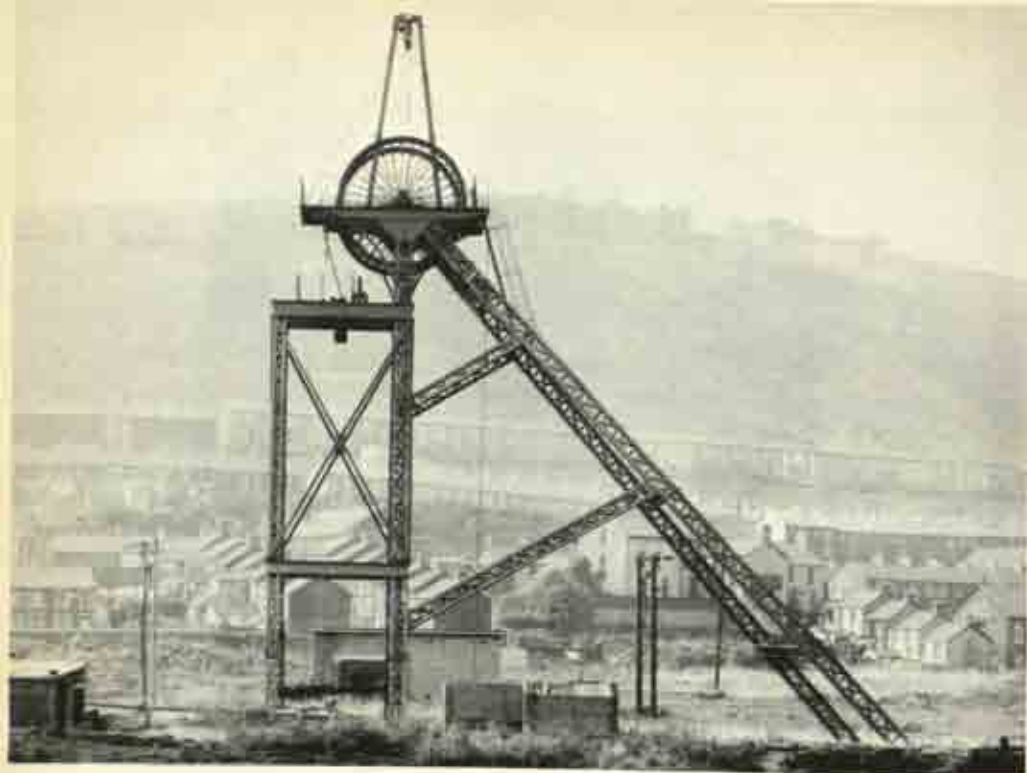
20 Cymcynon Colliery, Mountain Ash, Glamorgan. A typical late nineteenth-century headgear, now demolished
