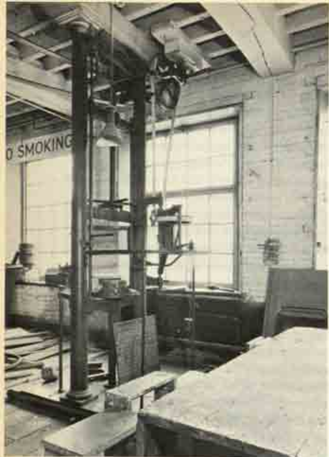
31 Saw at Portsmouth naval dockyard for cutting lignum vitæ. Installed in 1804 as part of Sir Marc Brunel's set of blockmaking machines
