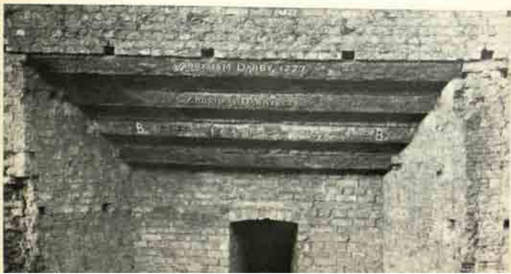
23 Abraham Darby blast furnace, Coalbrookdale, Shropshire. Detail of beams over forehearth
