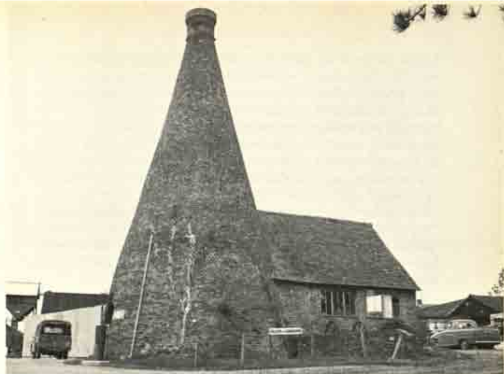
40 Conical brick kiln, Nettlebed, Oxfordshire
