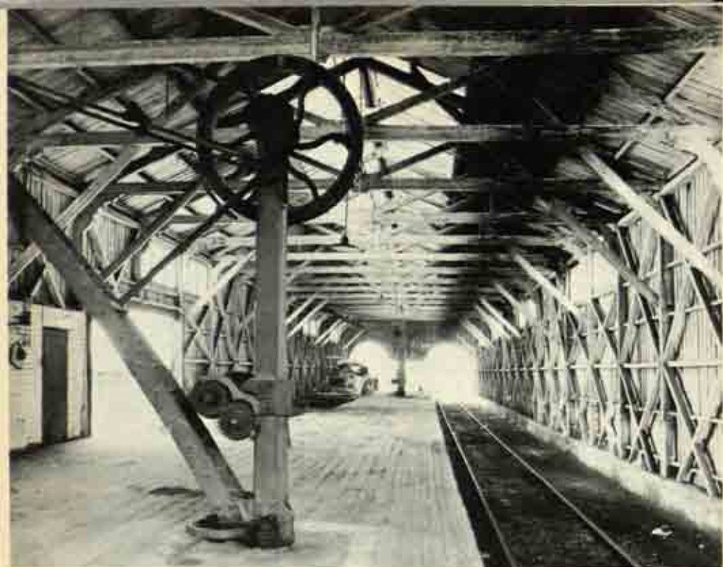
89 Great Western Railway broad-gauge standard-gauge goods transfer shed, Didcot, Berkshire
