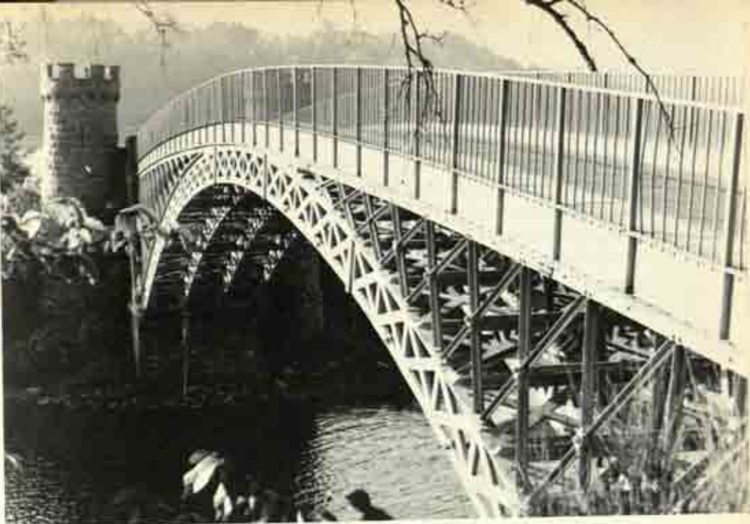
70 Thomas Telford's cast-iron bridge of 1814 across the River Spey at Craigellachie, Banff
