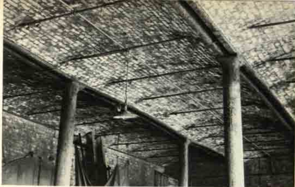
97 Albert Dock, Liverpool. Interior of warehouse showing cast-iron columns and beams with brick vaulting
