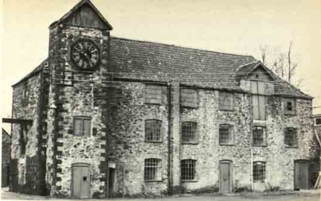
32 Warnley brass works near Bristol. The most substantial relic of William Champion's eighteenth-century works is this stone building incorporating black copper slag blocks
