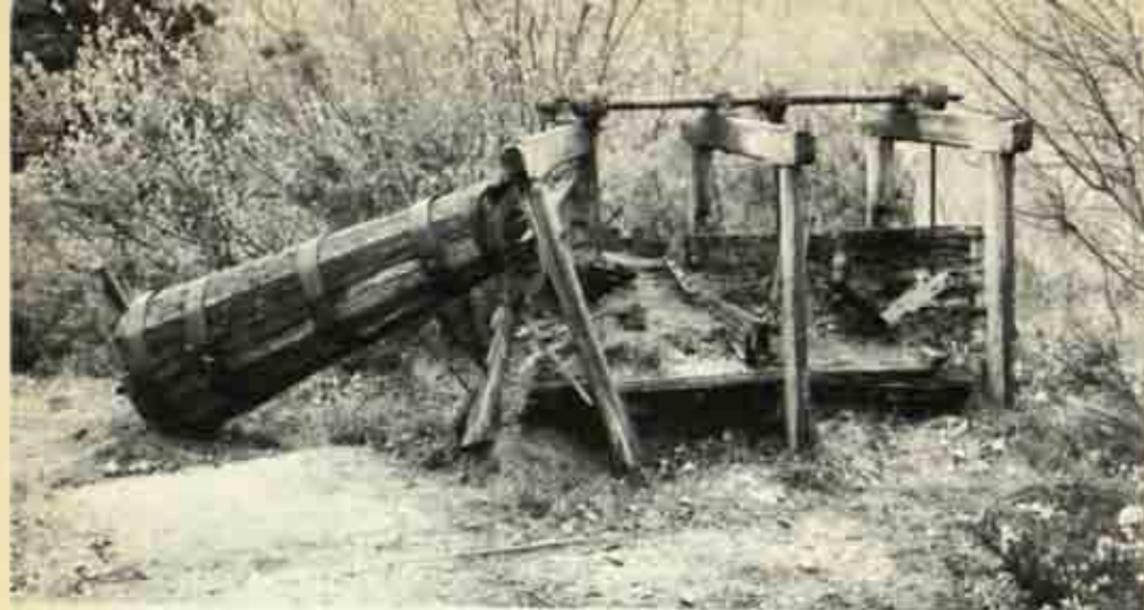
35 Snailbeach lead mines, Shropshire. Remains of ore separator with archimedean-screw feed
