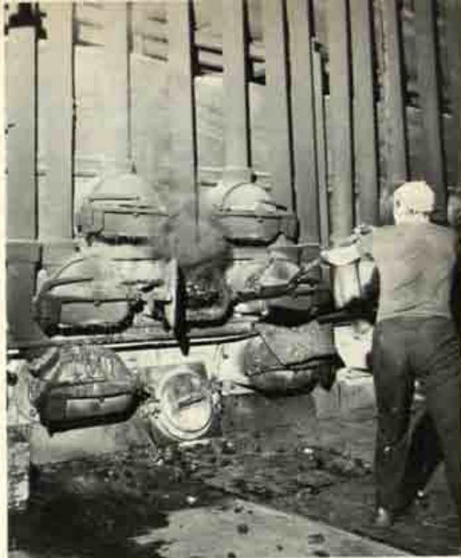
60 Hand-firing retorts at Girvan Gasworks, Ayrshire
