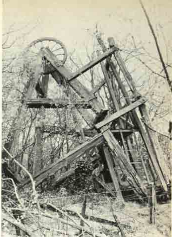
34 Snailbeach lead mines, Shropshire. Collapsed timber headgear
