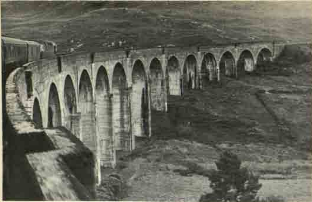
90 Mass-concrete viaduct at Glenfinnan on the Mallaig extension of the West Highland Railway, 1898
