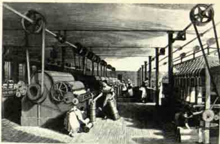
Fig. 29 Carding, drawing and roving (from The Circle of the Sciences , Vol II, 608)
