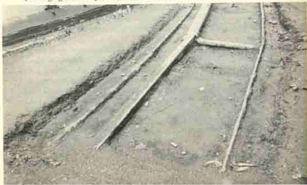
83 Dual-gauge cast-iron plateway, Coalbrookdale, Shropshire
