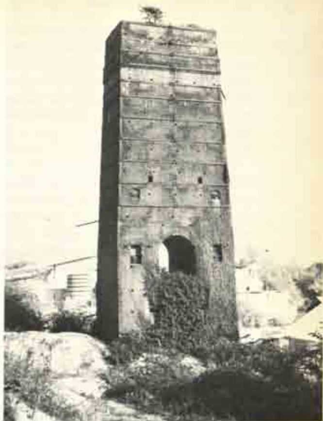
42 Split-shaft limekiln, 70ft high, at Betchworth, Surrey
