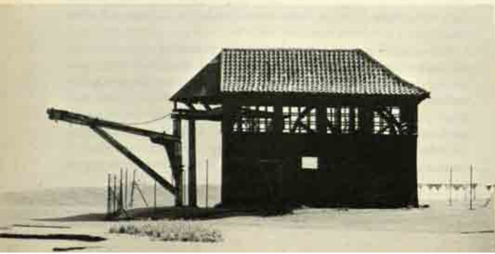
100 Treadmill-powered seventeenth-century quayside crane preserved at Harwich, Essex
