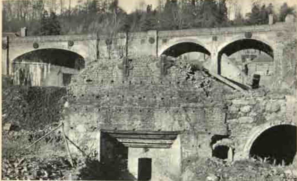
22 The blast furnace in Coalbrookdale, Shropshire, where Abraham Darby perfected the technique of smelting iron ore with coke in 1709. Excavation of the furnace site in the late 1950s
