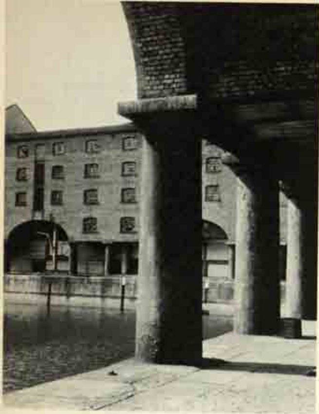
96 Albert Dock, Liverpool. Colonnade with cast-iron columns
