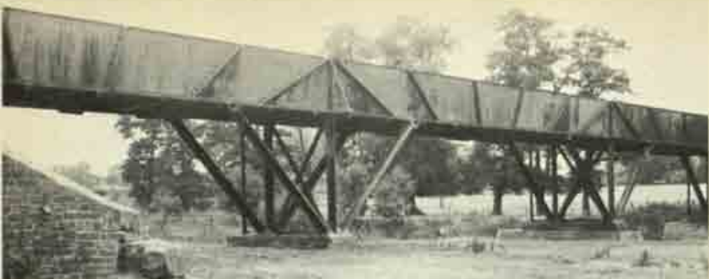
80 Longdon-on-Tern Aqueduct, Shropshire, by Thomas Telford. The first iron aqueduct in the world, built in 1796
