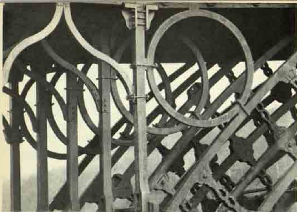
68 The Iron Bridge. Detail of arch showing dovetailing of radial members into ribs
