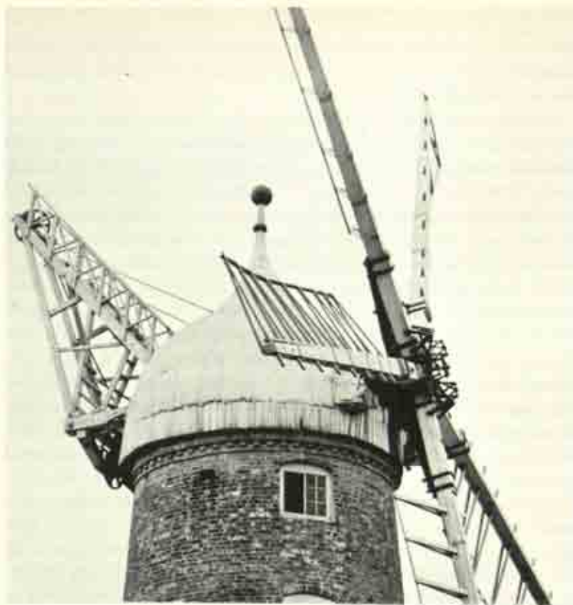
3 A tower mill: detail of the cap of the five-sail Maud Foster Mill, Boston, Lincolnshire
