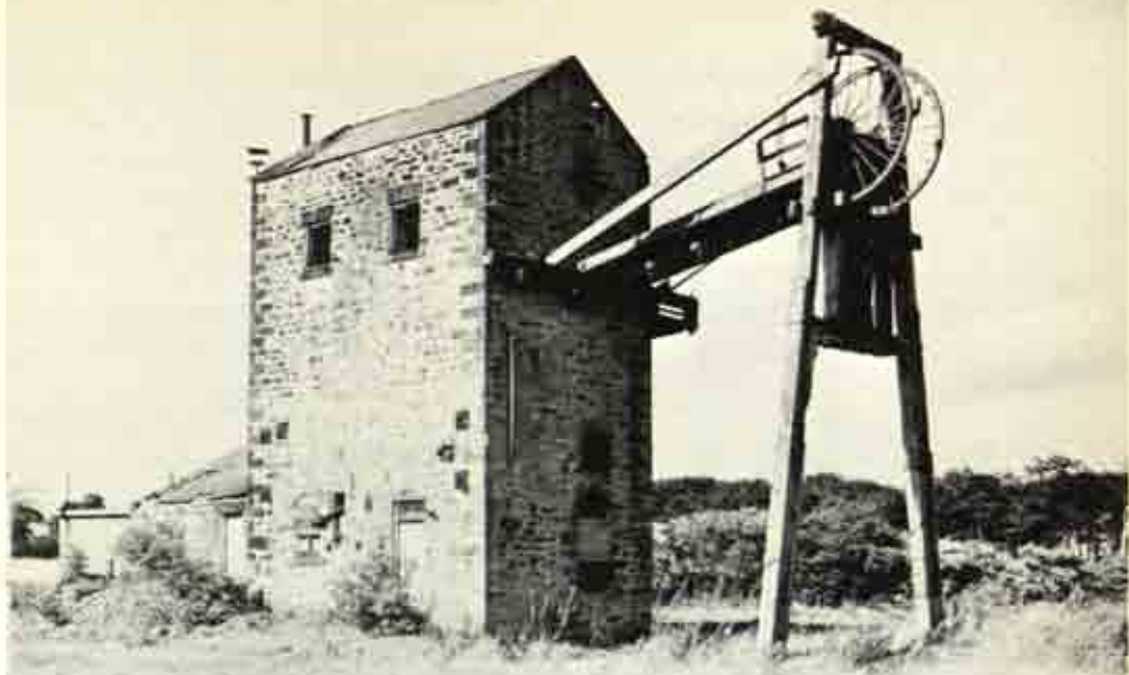
19 Beamish Colliery, County Durham. Winding engine-house and headstock, 1855
