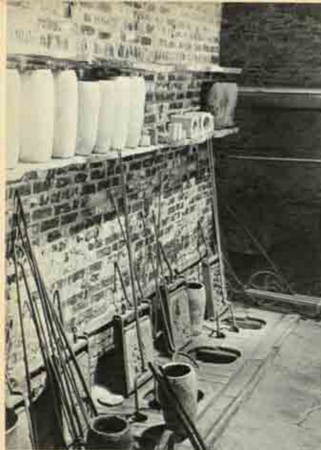
29 Crucible steel furnace, Abbeydale, Sheffield
