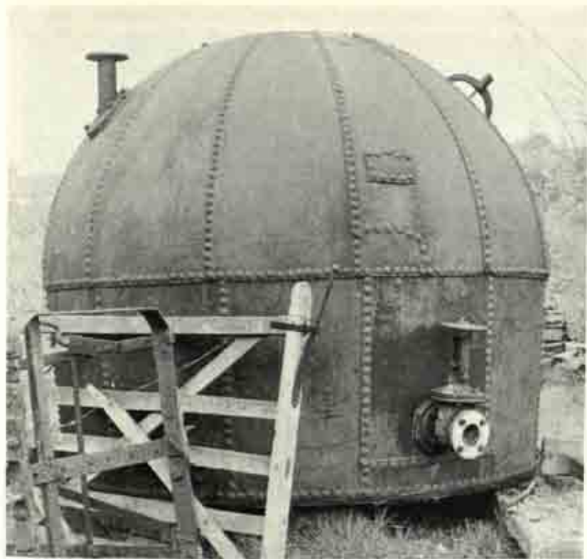
14 Haystack boiler, Blists Hill Open Air Museum, Ironbridge, Shropshire
