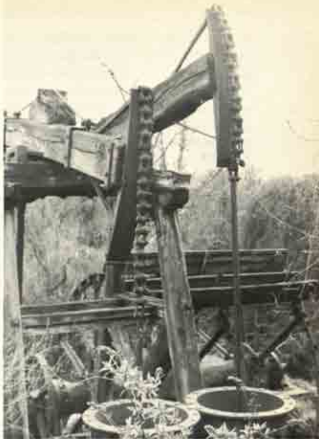
33 Melingriffith water pump, Glamorgan. Double-beam pump powered by an under-shot waterwheel and used to return water from the River Taff to the Glamorgan Canal
