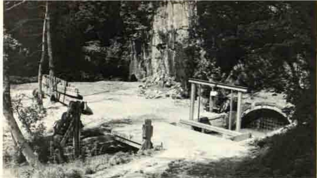
21 Entrance to the coalmines at Worsley, Lancashire. On the left is a 'starvation' boat used on the underground canal system
