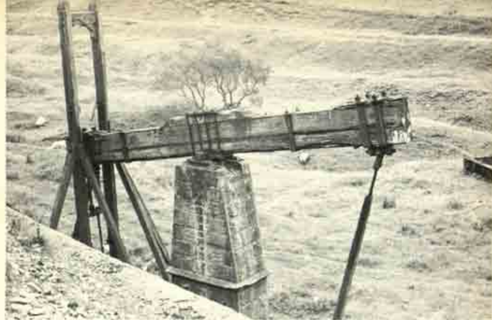
37 Water bucket beam engine at Straitsteps lead mine, Wanlockhead, Dumfriesshire
