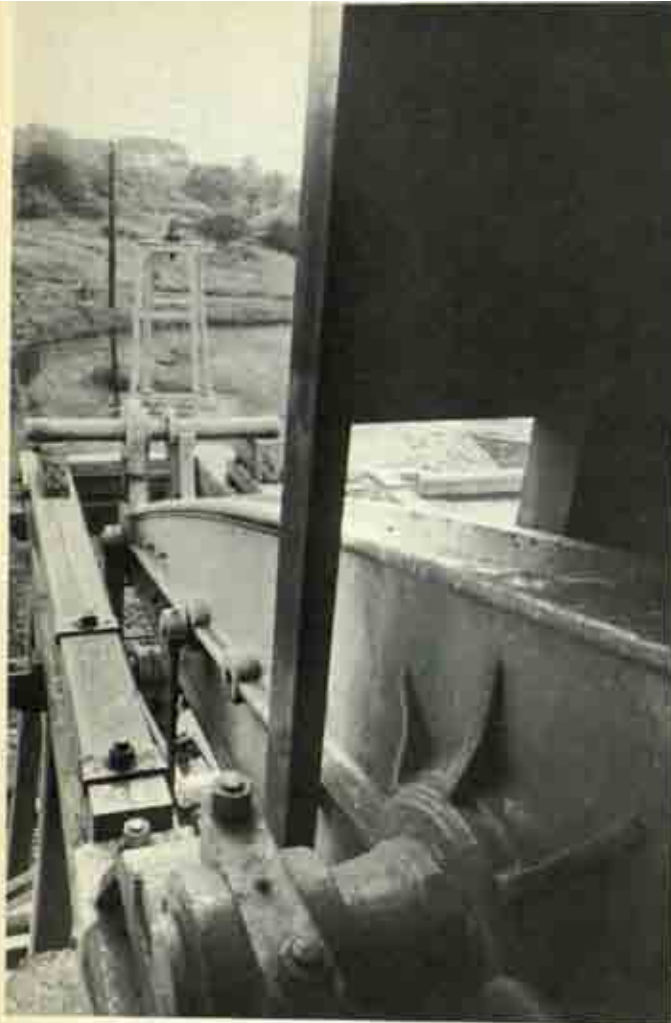
9 Elsecar beam engine. Detail of cast-iron beam
