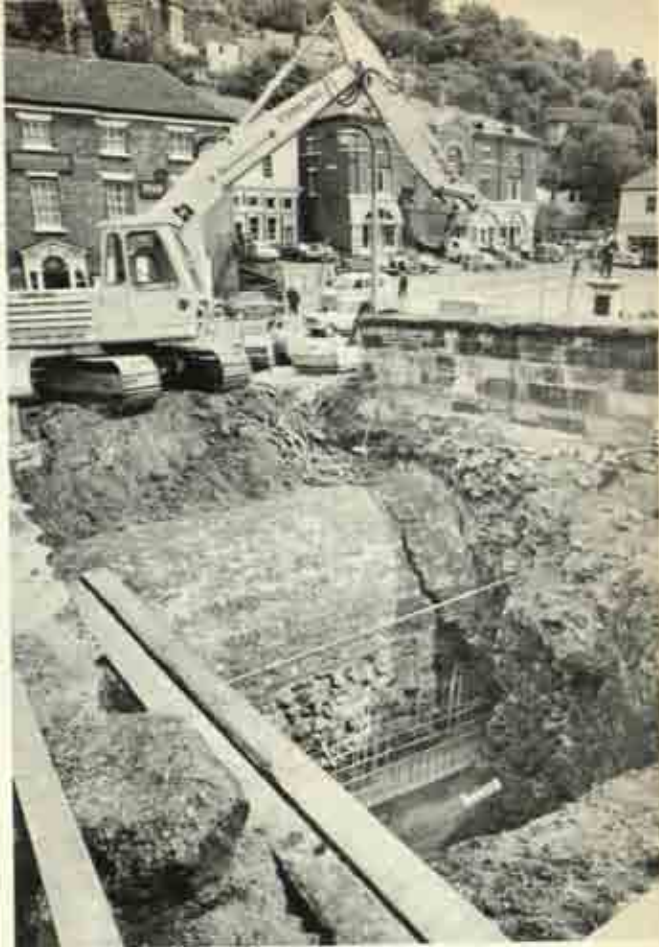
69 Restoration of the Iron Bridge. Excavation of the north abutment and insertion of reinforced concrete strengthening
