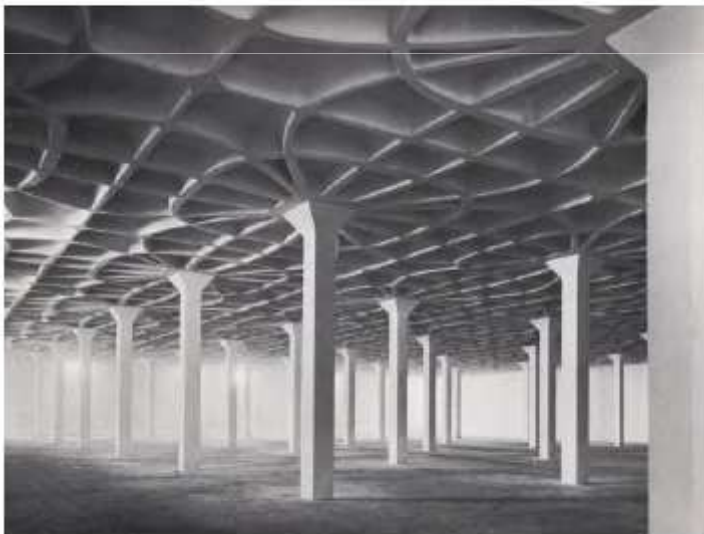
Fig. 4. Gatti Wool Factory Floor System [13]
