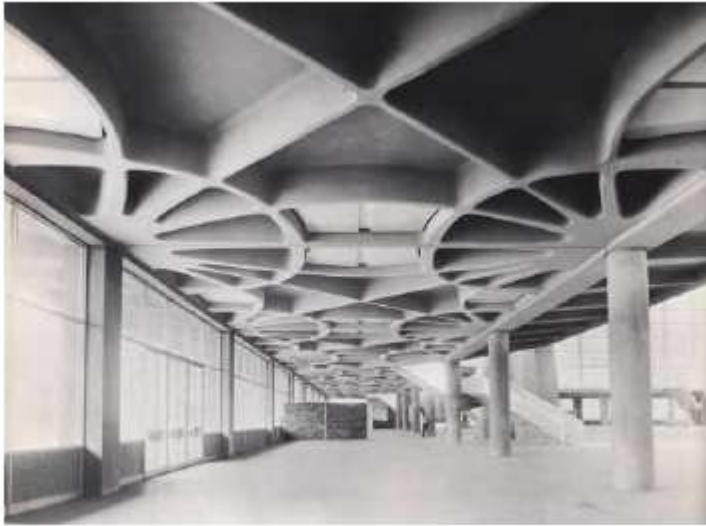
Fig. 7. Palace of Labor Floor System [13]
