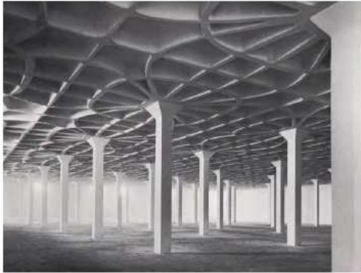
Fig. 4. Gatti Wool Factory Floor System [13]
