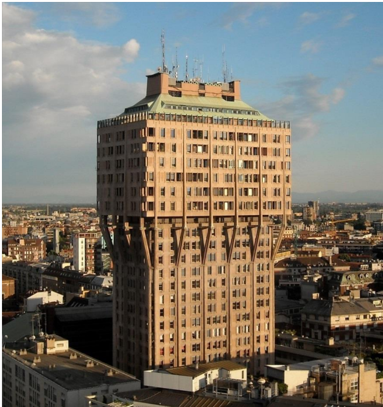
Studio BBPR, Torre Velasca, Milano (1957)
