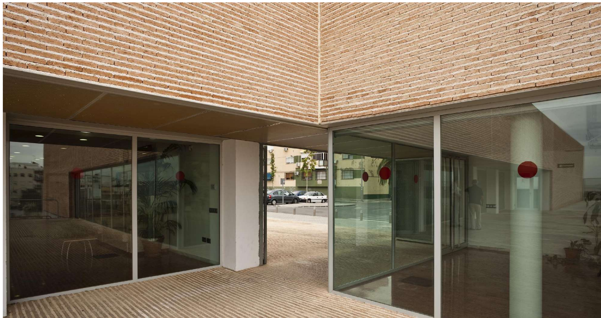
JAVIER HARO GREPPI, DAY CARE CENTRE IN ALCALÁ DE GUADAIRA
