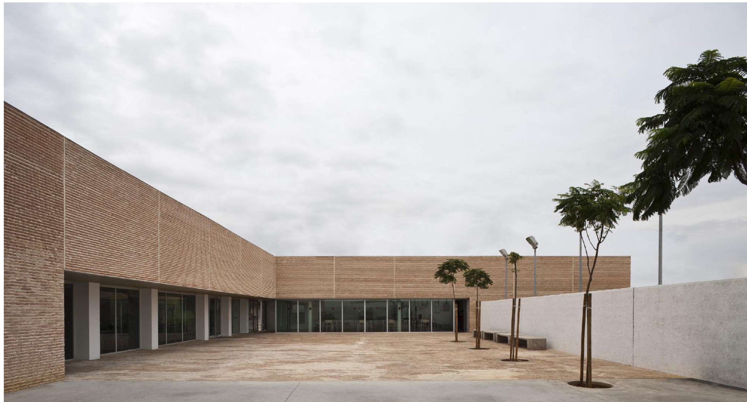
JAVIER HARO GREPPI, DAY CARE CENTRE IN ALCALÁ DE GUADAIRA
