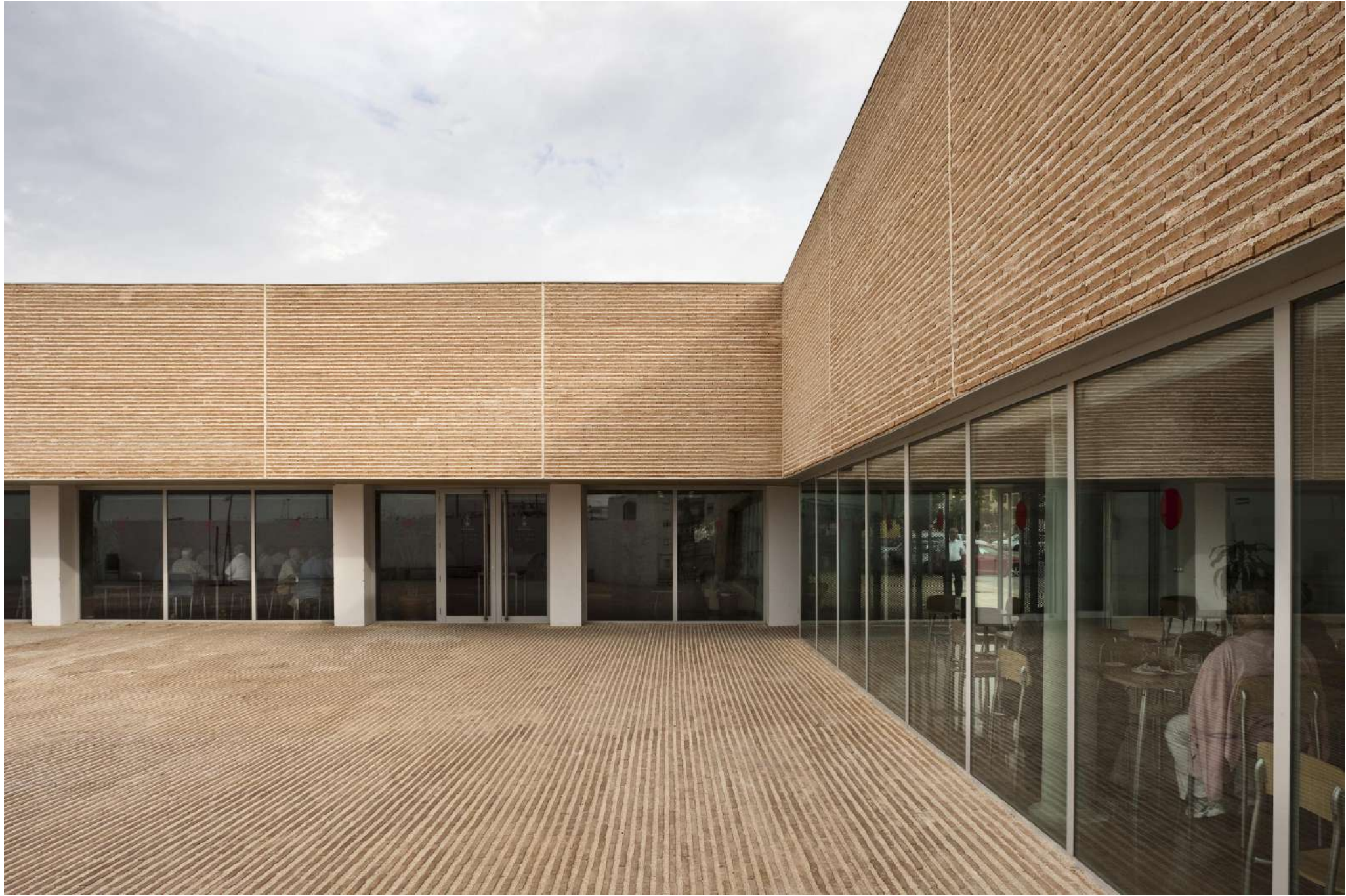
JAVIER HARO GREPPI, DAY CARE CENTRE IN ALCALÁ DE GUADAIRA
