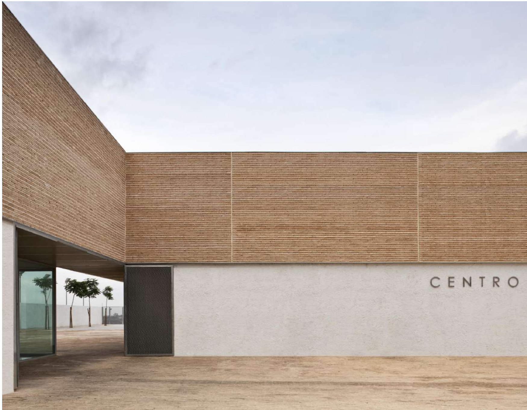
JAVIER HARO GREPPI, DAY CARE CENTRE IN ALCALÁ DE GUADAIRA
