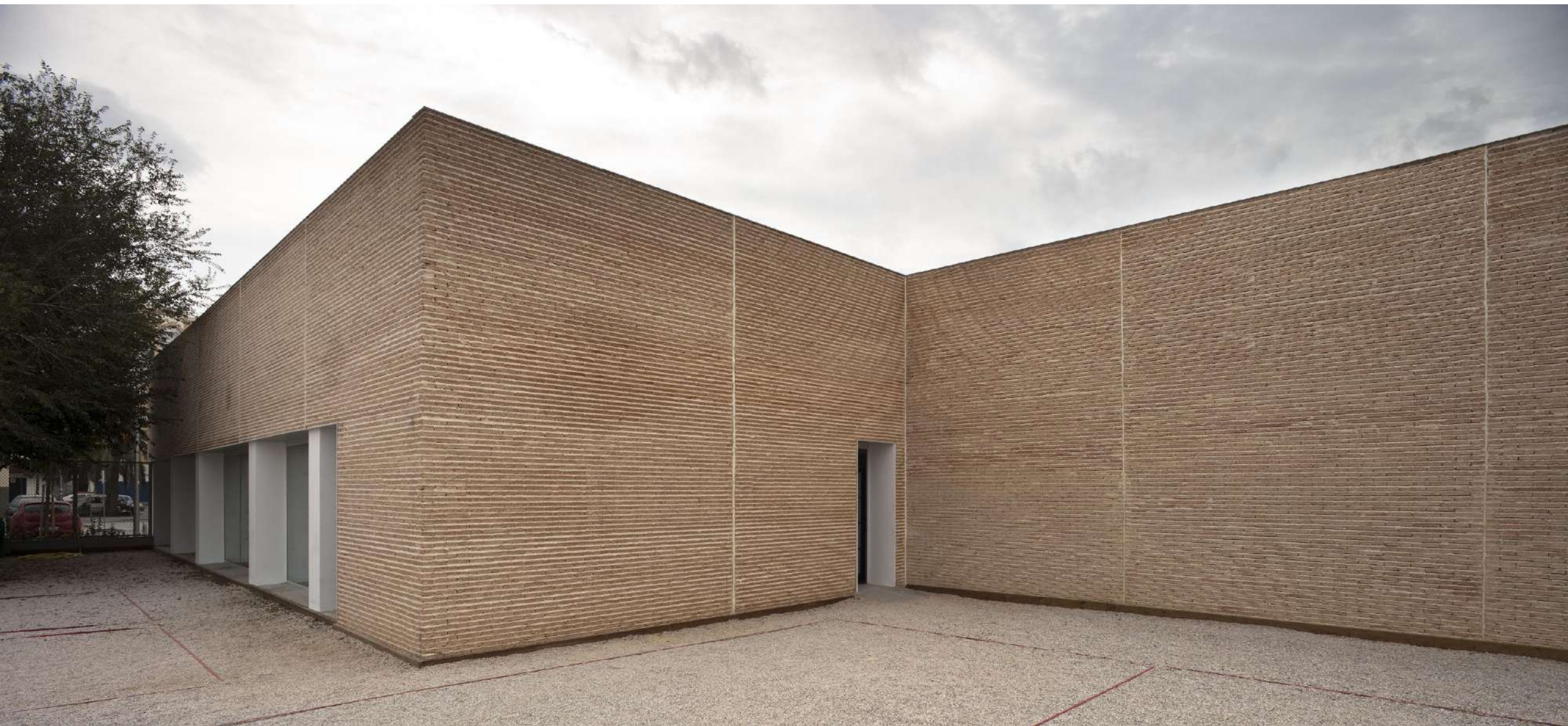
JAVIER HARO GREPPI, DAY CARE CENTRE IN ALCALÁ DE GUADAIRA
